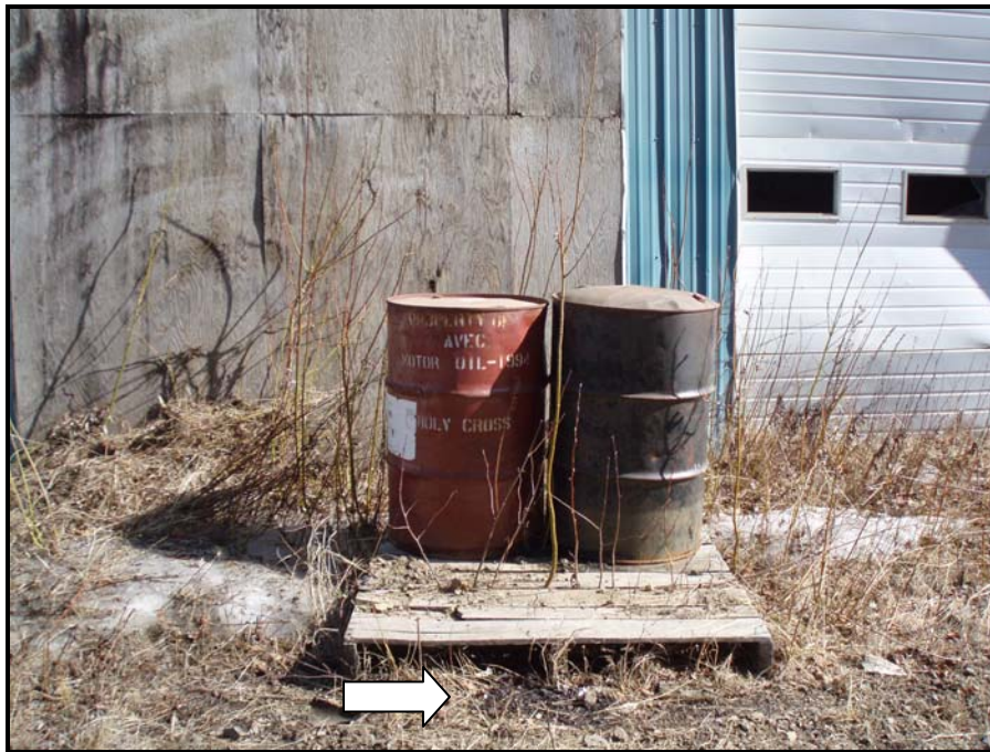
Photograph 9: Close up of 55-gallon barrels in front of City Shop. The black barrel is bulging and stained soil can be seen in front of the pallet (see arrow).
